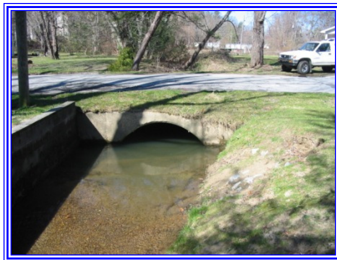
Figure 7.7: Meadowbrook Terrace Culvert.
