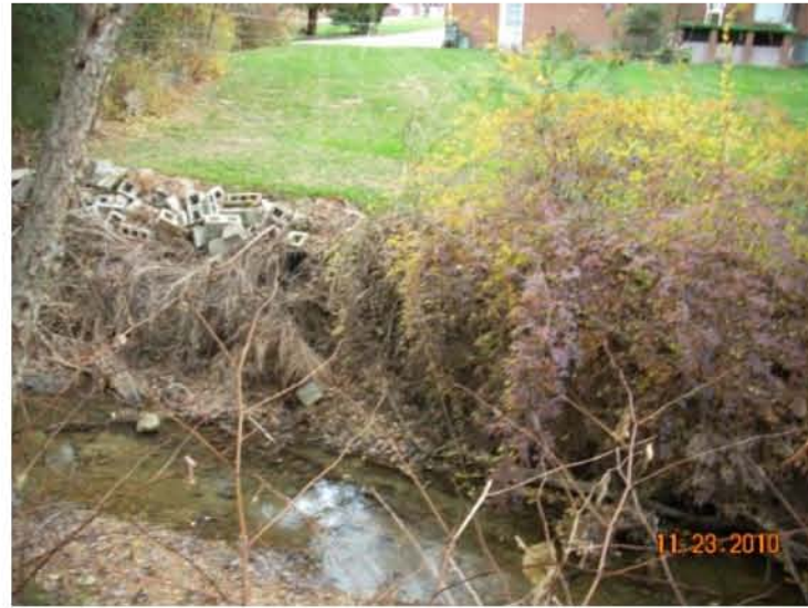
TRIBUTARY 2 DOWNSTREAM OF NORTH HARPER DRIVE
