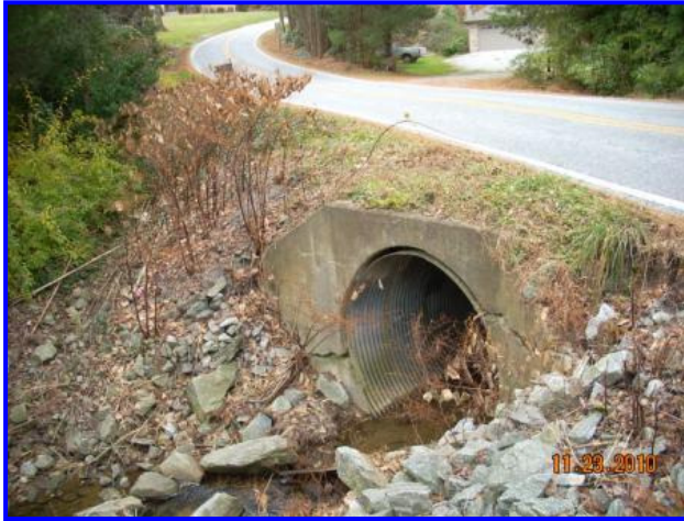
Figure 5.9: Headwall Browning Avenue.
