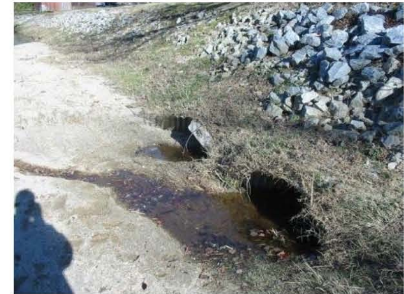
BRITTON CREEK JUST DOWNSTREAM OF ASHEVILLE HIGHWAY
