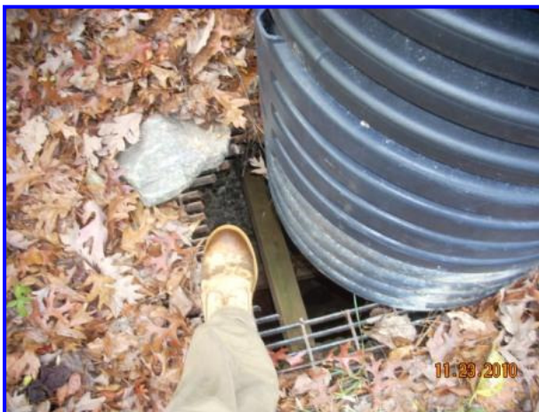
Figure 5.11: Open Grate Inlet Burke Lane.
