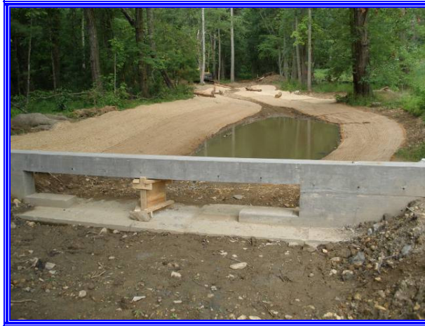
Figure 7.11 Dingle Creek during construction
