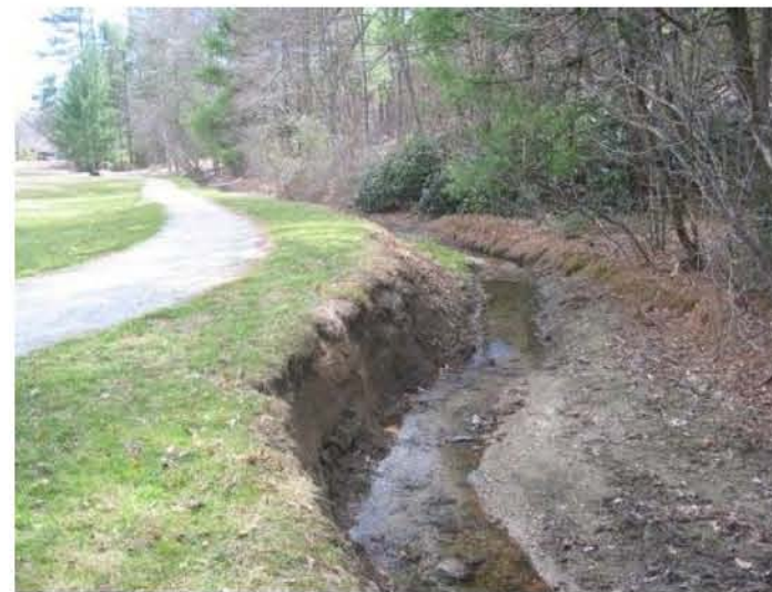
SMALL TRIBUTARY TO BRITTON CREEK NEAR 'THE OAKS'
