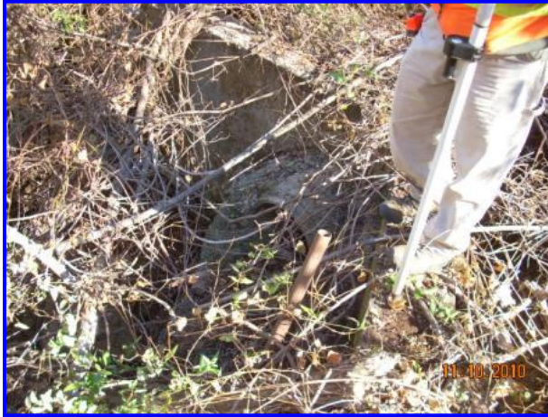
Figure 5.7: Headwall at Hendersonville Elementary.
