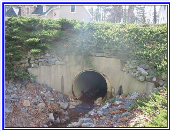
Figure 7.1: Enclosed Culvert (Mistletoe Trail)
