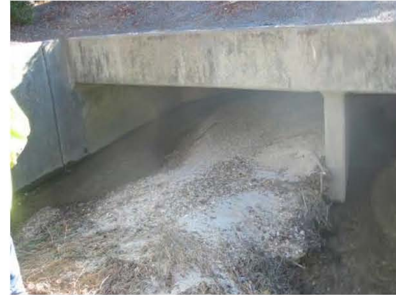
BRITTON CREEK JUST DOWNSTREAM OF ASHEVILLE HIGHWAY
