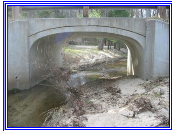
Figure 7.2: Bottomless Culvert (Maplewood Court)
